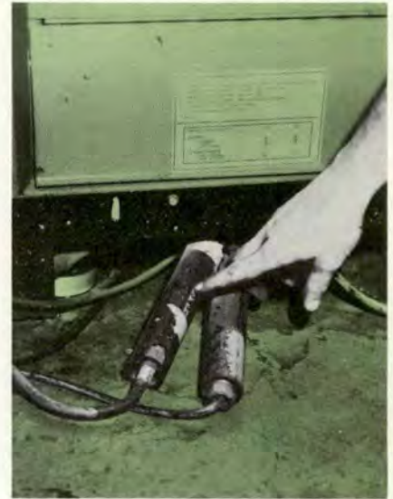
Poor example! Heliarc fuses should be properly shielded and mounted to prevent damage, assure easy access.
